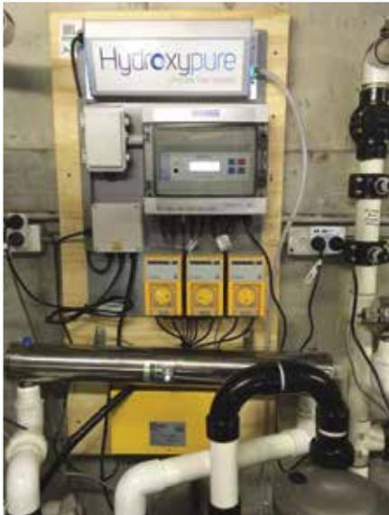
*The Hydroxypure system continually sanitises your swimming pool by testing the water and automatically maintaining optimum levels of residual sanitiser.*
