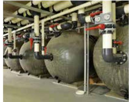
*Waterco's Micron commercial filters have received certification to NSF/ANSI Standard 50. Its certification verifies compliance with the American National Standard for confirming performance, safety, and material health effects requirements have been met. Most American commercial pool codes require compliance with NSF/ANSI Standard 50.*
